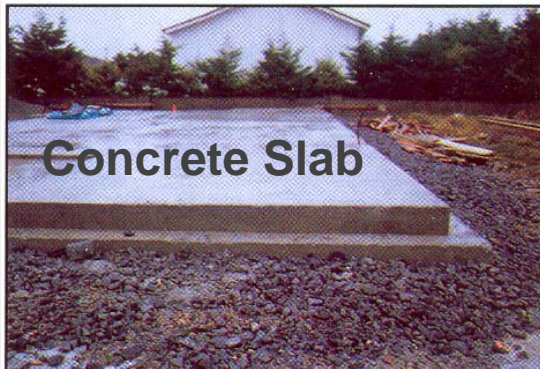
Fig 1 : Raft foundation
